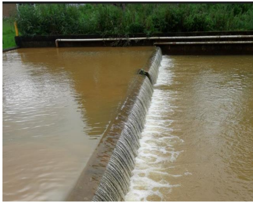
Figure 2. Sedimentation pond for production of ochre sludge. From vudp.dk
